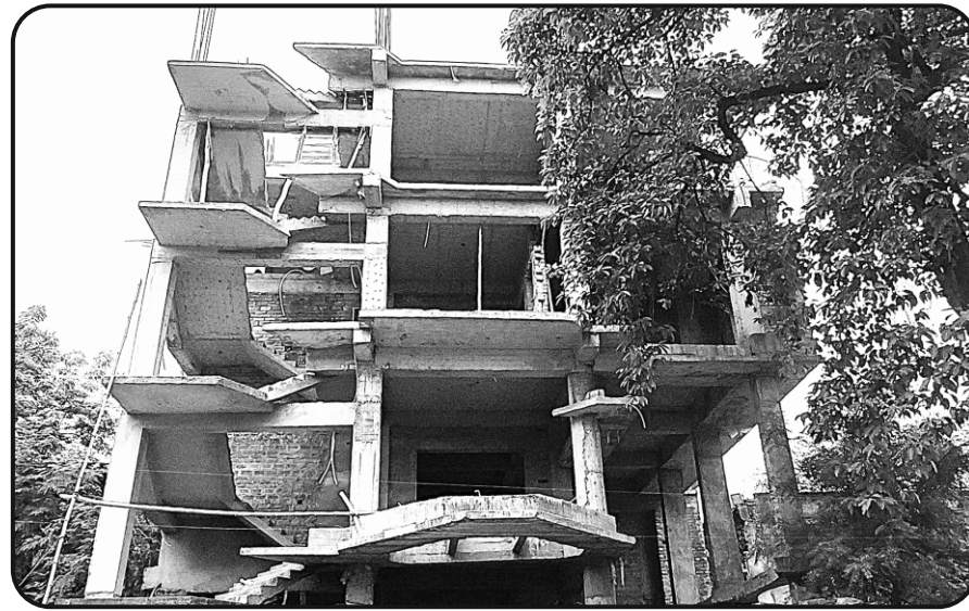
The above picture of ongoing construction work of the School Building in a prominent place (At 28A/6, Ratanbabu Road, Kolkata - 700002) for free education facilities mainly to the slum children
